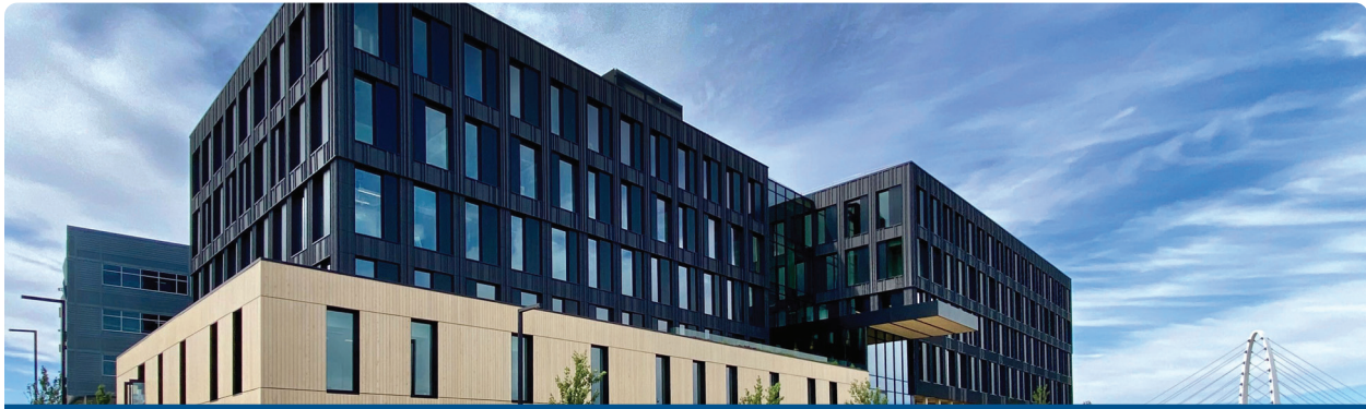
EWU Catalyst Building in Spokane, WA
