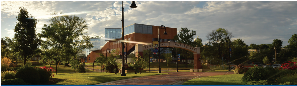
Kent State University Campus Entrance View
